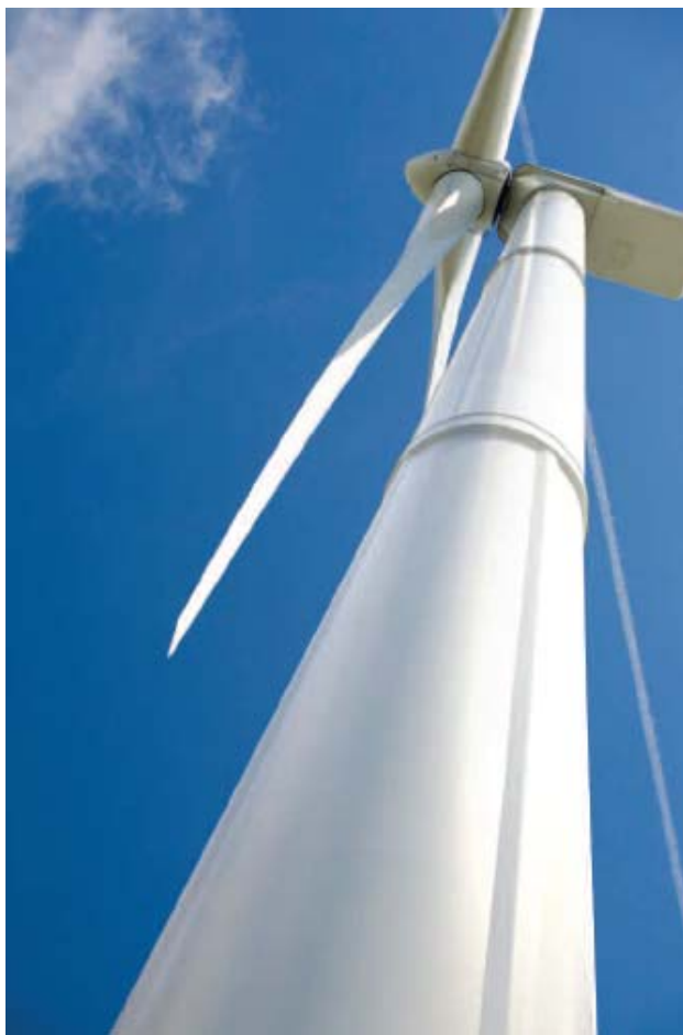
Figure 9. Wind turbine tower produced by Northstar, with bolted friction joints both in longitudinal and lateral directions.
