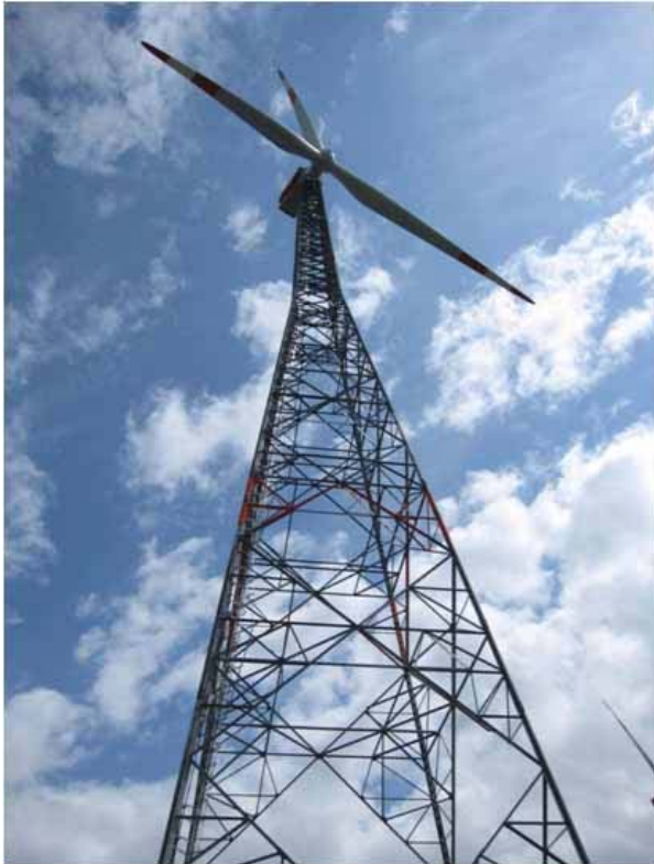
Figure 20. A Fuhrländer 2,5 MW wind turbine with 100 m turbine diameter and a lattice tower providing 141 m hub height. Photo Vattenfall.
